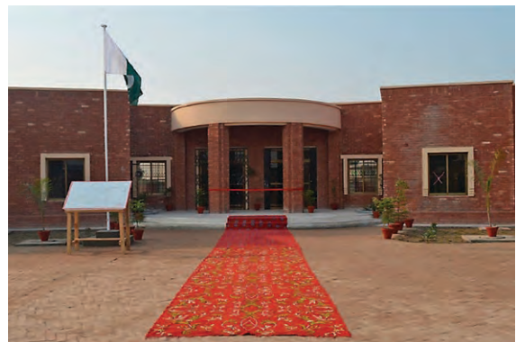
> Figure A12: Khanki girls' high school. Entrance to the new building located in Khanki Village.
