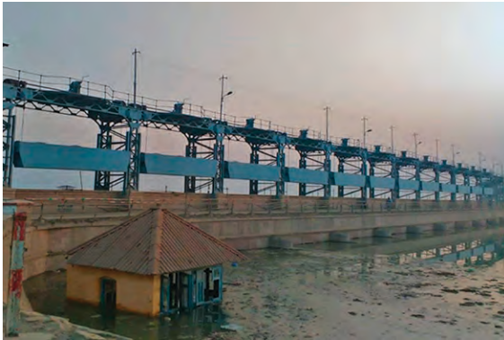
➤ Figure A1: The Old Khanki Headworks. One of the oldest headworks in Pakistan, completed in 1892 and dismantled in 2016.
