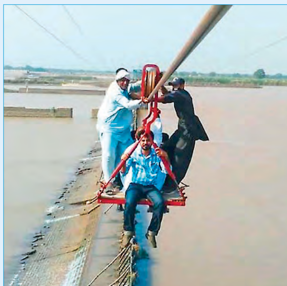
➤ Old Practices. Workers used the trolley for operations and maintenance in dangerous conditions at the old Khanki Headworks (photo by the Project Management Office Barrages, Punjab Irrigation Department).
