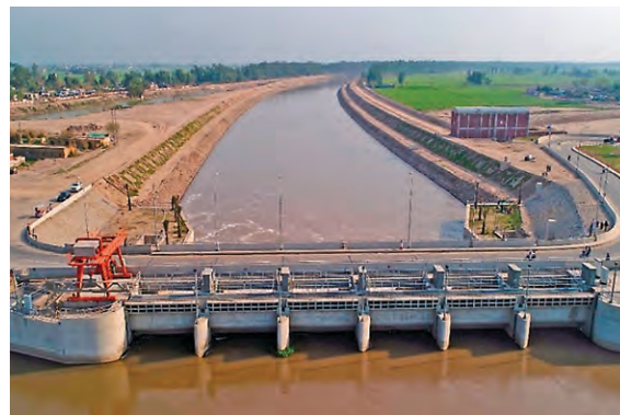
➤ Figure A6: The new Lower Chenab Canal headwork. The new headworks replaced the 120-year-old structure.
