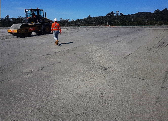
Figure 22 Rubblisation of concrete pavement, Varsity to Tugun, QLD
