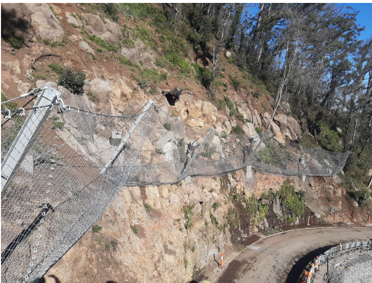
Figure 23 Rock fall netting installed at Binna Burra
